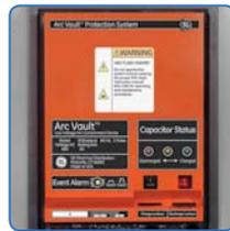
When activated, Arc Vault continuously monitors current and voltage to identify an arc flash.
